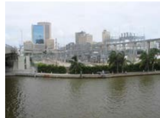
Existing: FPL Substation
